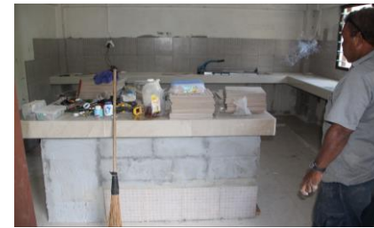
Photo 6: The wet lab under construction for biological sampling at NFMRA
